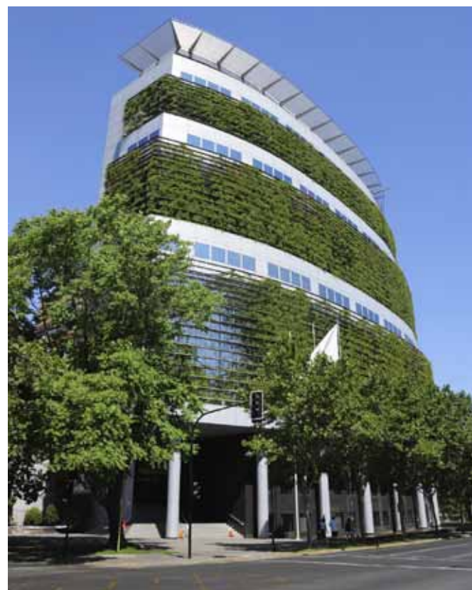
Foliage helps cool this building in Santiago, Chile.
