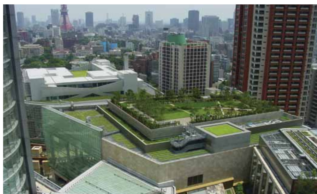
By incorporating green roofs and urban parks a city can effectively reduce the "heat island" effect.
