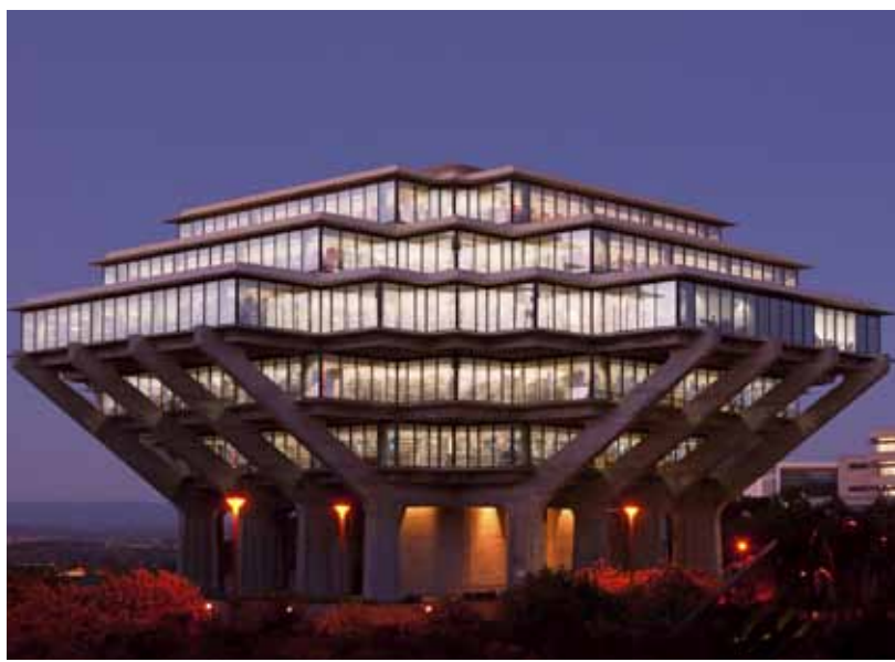
The University of California San Diego is a test-bed for smart grid innovations that can permit real-time, two-way flows of power and digital information.
