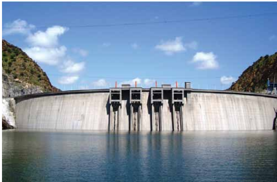
The Tekeze Arc Dam, one of the hydro plants completed in 2009, generates 300 MW.
